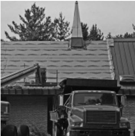
church roof repairs
