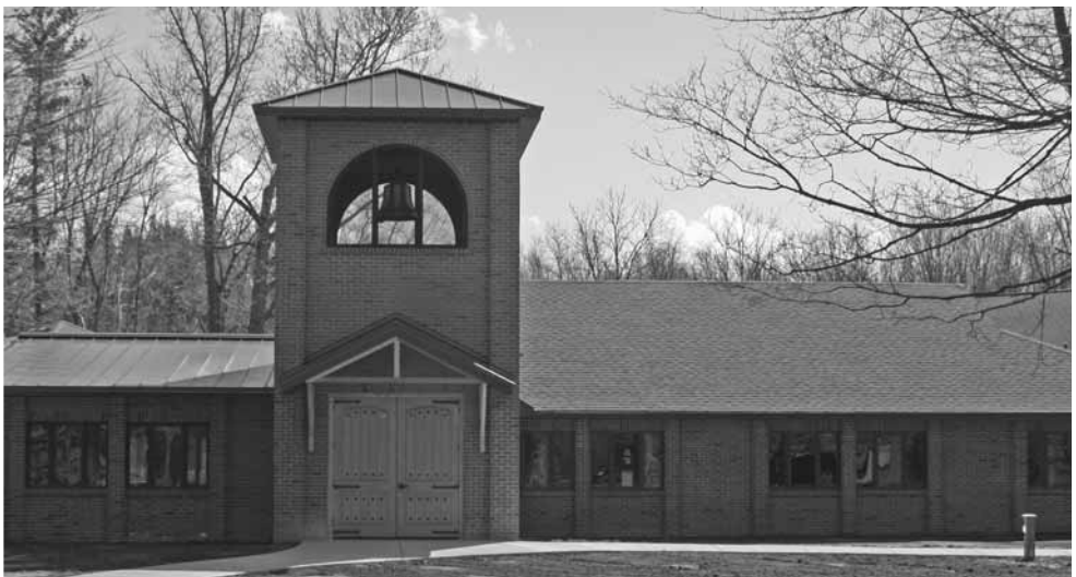
the new church entrance and bell tower
