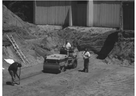
preparing the ground for the new building
